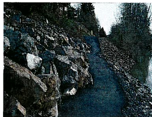
Existing trail at repair site
