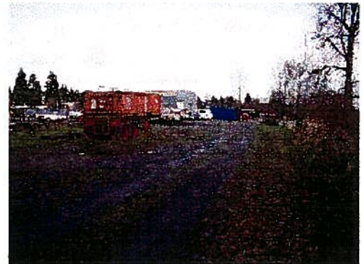
Public Works Shop site
