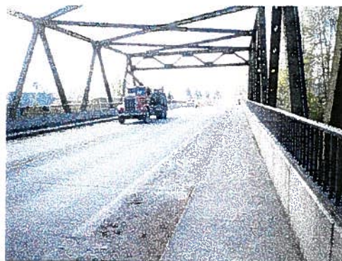
Avenue D bridge
