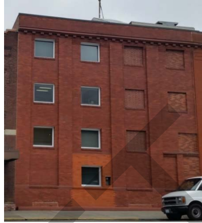
Original windows have been bricked over.
