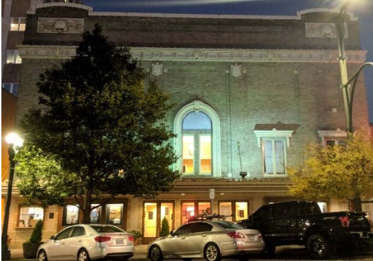
Exterior light fixtures that emphasize architectural elements.
