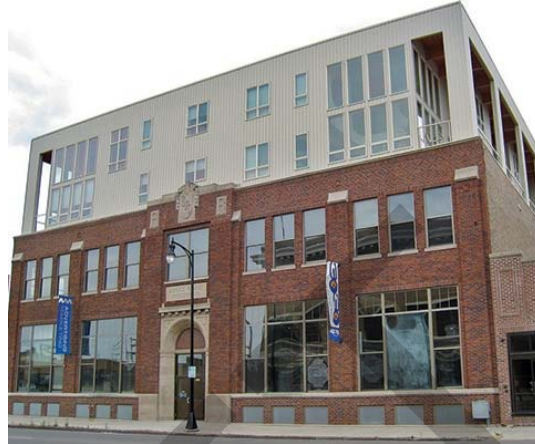
Addition above roof of historic building becomes a focal point with inappropriate materials.
