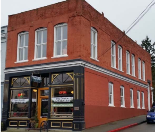
Vertically-oriented windows with true muntins have been maintained.
