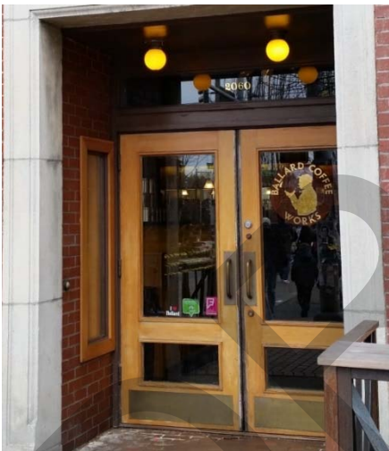
Wood doors with extensive glazing, kick plates and bronze hardware.
