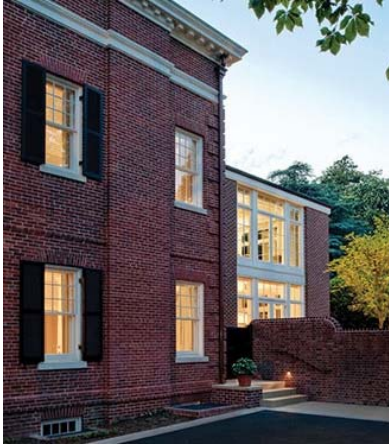
Addition to the rear of an historic building uses similar materials without creating false sense of history.
