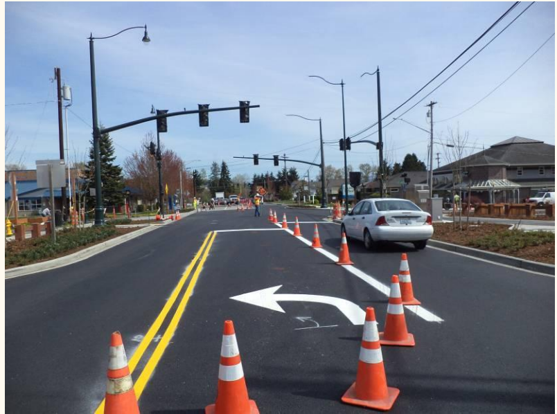
View looking east from Second Street, just west of Lincoln Avenue
